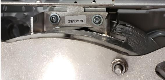
Fig. 11: Heat Exchanger Bracket Screws
